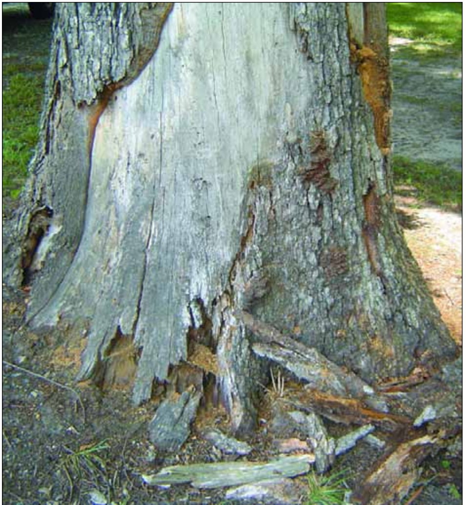
Slime was seen fluxing here in 1998, but it was untreated. Removal is now required.
